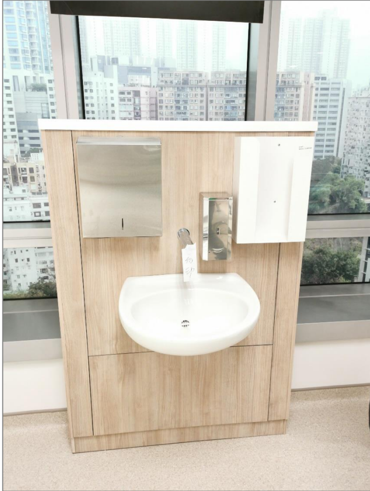
Kwong Wah Hospital, Ongoing
