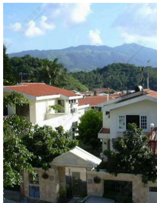
Hong Lok Yuen (Renovation)
